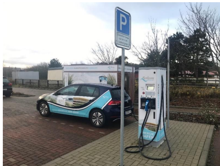
Figure 40 Charging station "Am langenWasser"
